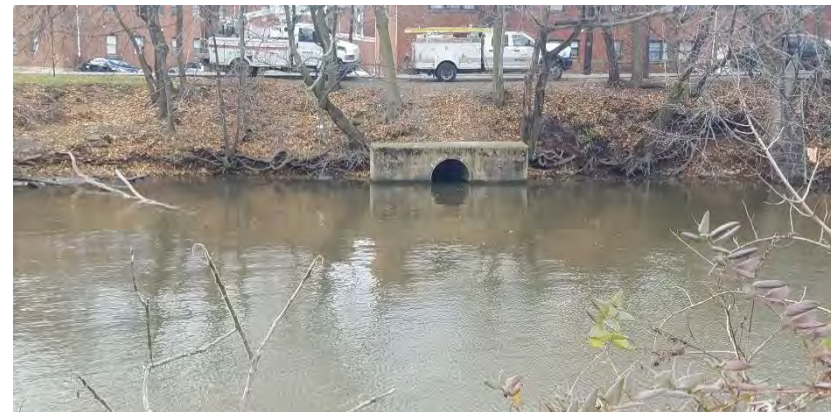
Existing Stormwater Outfall at Admiral's Cove
