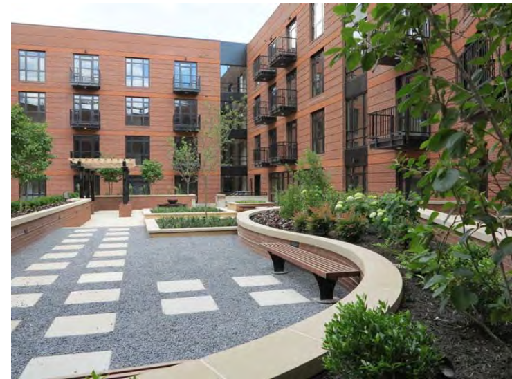
700 Constitution Apartments – rear façade – Washington, D.C.
