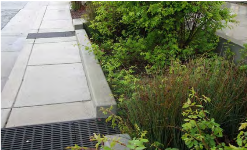
Urban Runoff Treatment Retrofit
