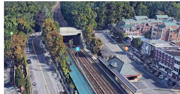
North Astor Street Rail Overpass Village of Irvington, NY Credit: Google Maps- October 23, 2019
