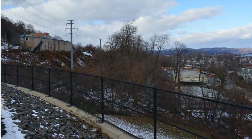
Haverstraw Transit Site with Slopes Apparent
