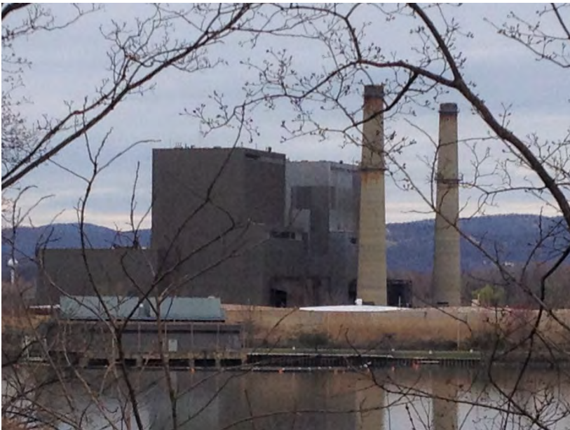
Bowline Generating Station
