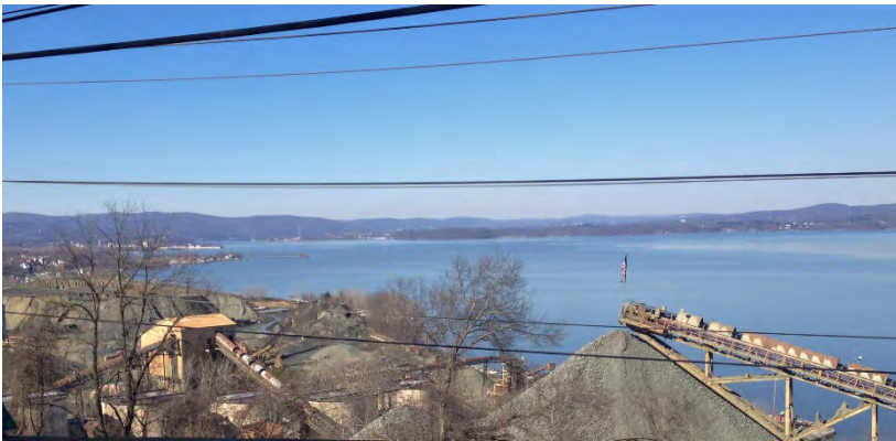
Tilcon Yards in the foreground looking towards the Hudson River Credit: Nautilus International, March 2019
