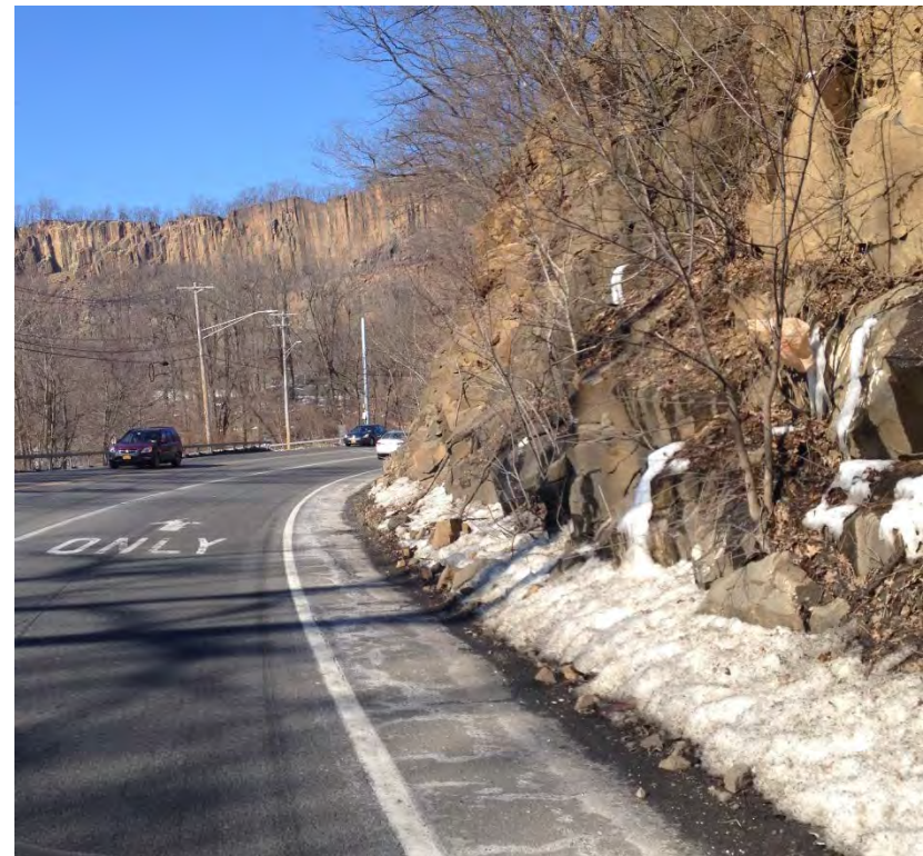
Route 9W approaching from the south
